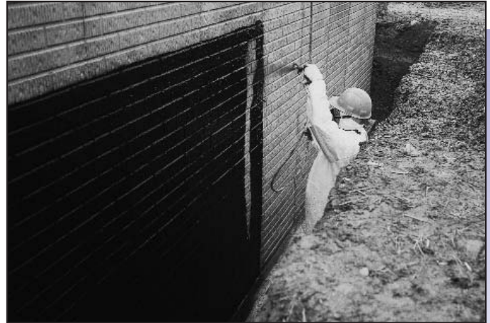
PolyPro Dampproofing is spray-applied for seamless coverage of foundation walls.
